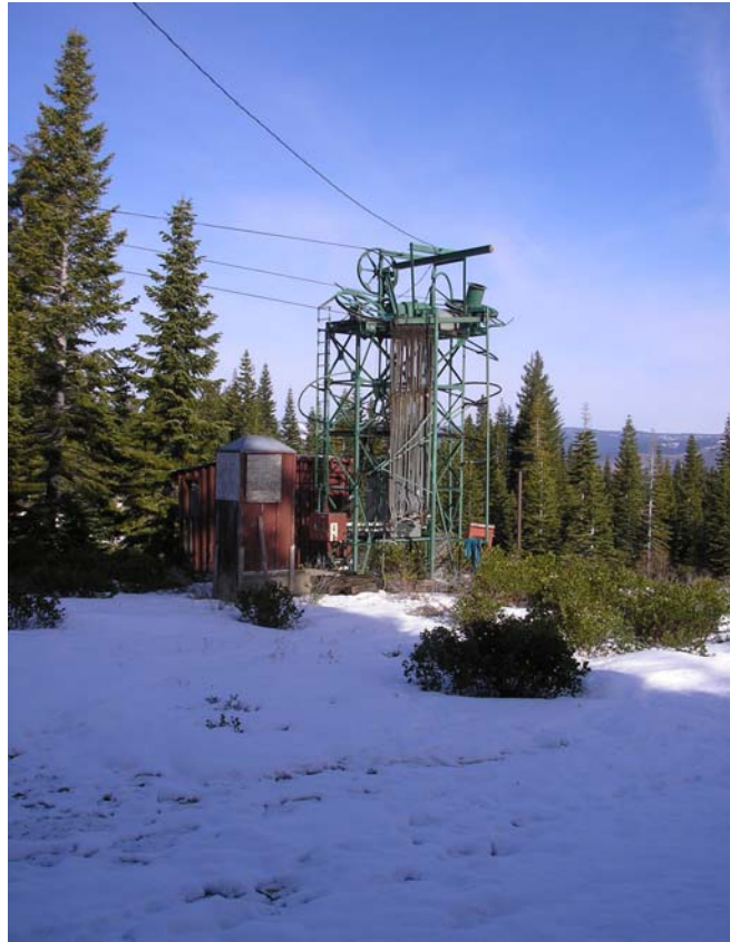
2 Old Poma Lift Infrastructure
